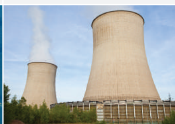
Nuclear / Power Stations
